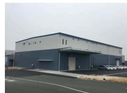
OHBA SEIKEN's new factory building
