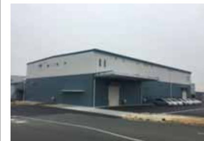
OHBA SEIKEN's new factory building
