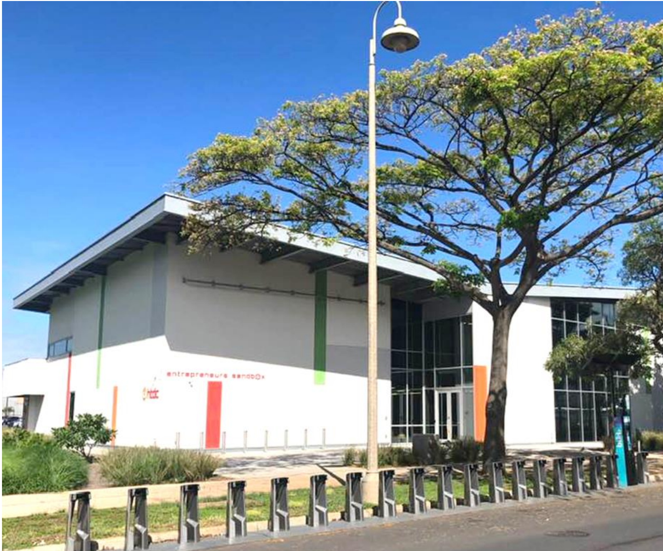
Note: fabbit occupies part of the building shown here.
