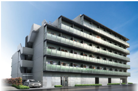
Genovia series exterior (Genovia Nerima-Takanodai skyrun)
