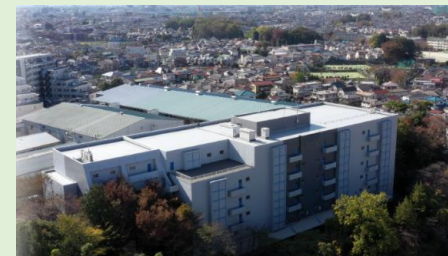
The 1st Tokyo Distribution Center
