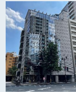
BIZIA Koujimachi Building
