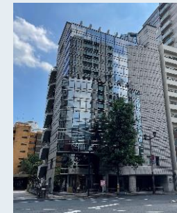
BIZIA Koujimachi Building
