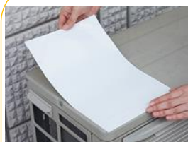
AC outdoor unit thermal insulation sealing
