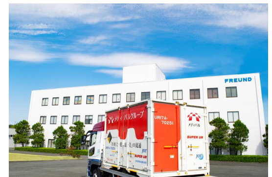
Top: Loading a container Bottom: A container at the Hamamatsu Factory
